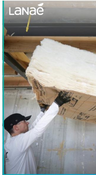
Glass wool containing up to 80% recycled materials and bio-based binder
